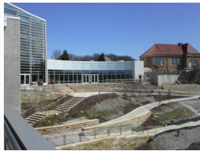
— Looking back from the green roof: the new landscaping (all with native plants) is visible, along with the older part of the conservatory in the background.
